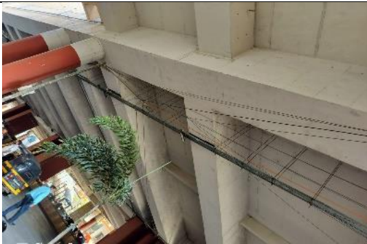
New painting at Road level had been done by MMRDA
