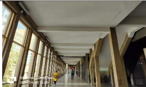
New Painting for the ceiling at Concourse level after CMRS Inspection.
