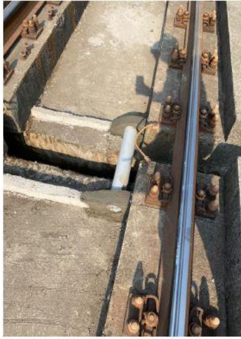
Inter connection of rain water diversion from one U- girder to adjacent U -Girder.
