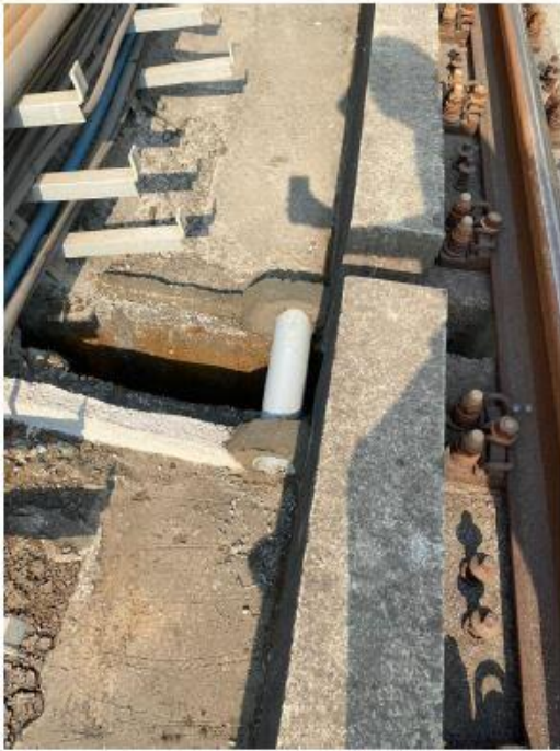
Inter connection of rain water diversion from one U- girder to adjacent U -Girder.
