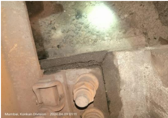
Repaired Baseplates Pedestal
