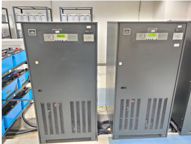
One Additional UPS installation
