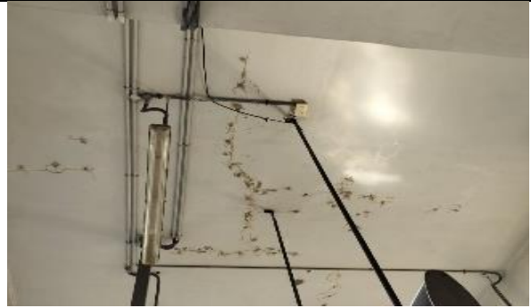
Injection Grouting patch observed near PD level slab
