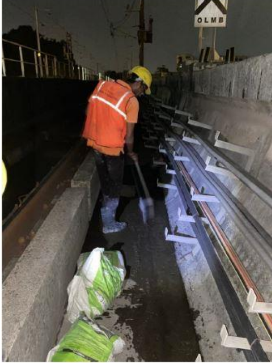
U-girder deck slab undulation leveling and slope correction work.
