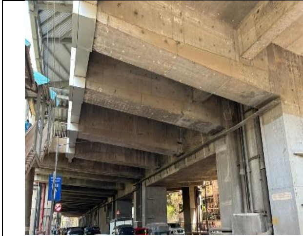
Anti-carbonation painting is pending in Road level.
