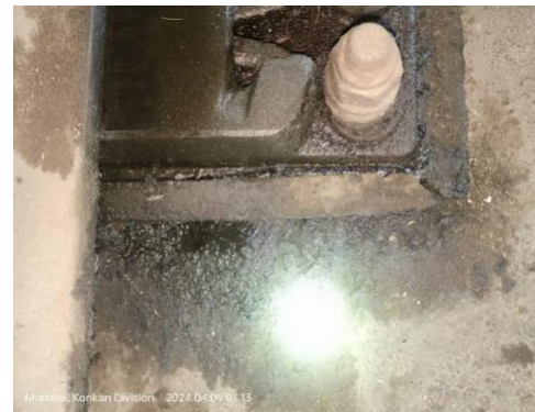
Repaired baseplates Pedestal
