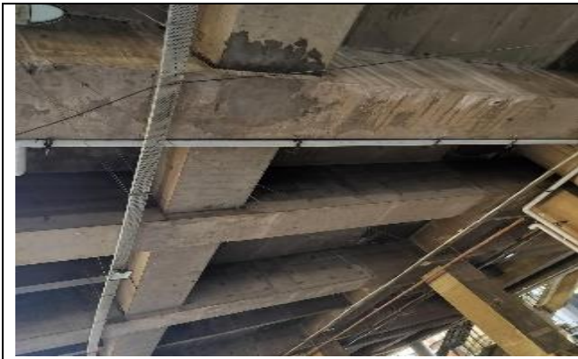
Anti-carbonation painting is pending on Road level
