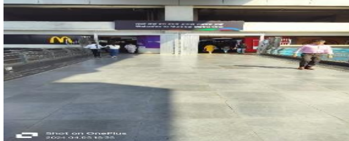
A New Opening was provided for the connection of FOB constructed by MMRDA which connects the Gundavali Metro Station
