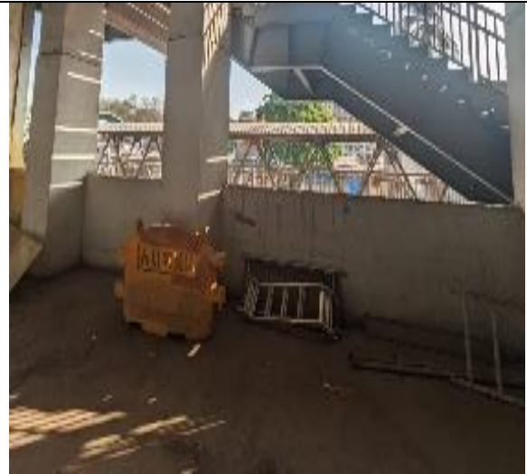
Emergency Stair provides for passenger evacuation during any incident.
