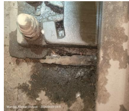
Repaired Baseplates Pedestal
