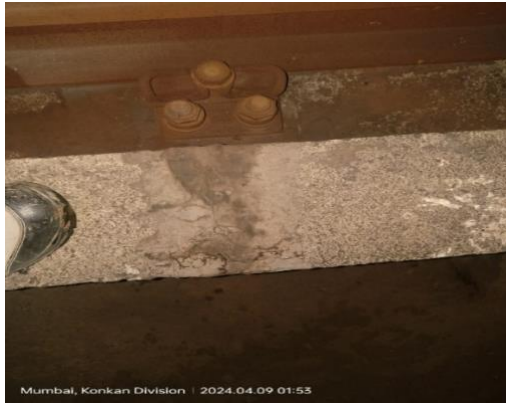
Repaired Derailment Guard
