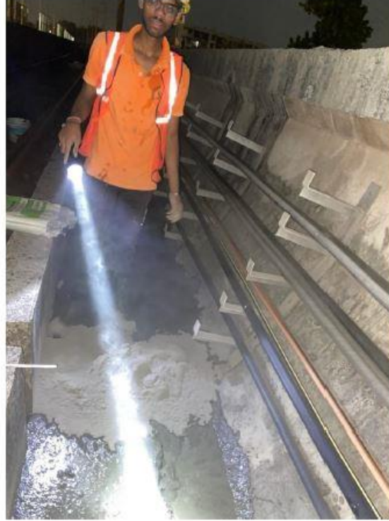
U-girder deck slab undulation leveling and slope correction work.
