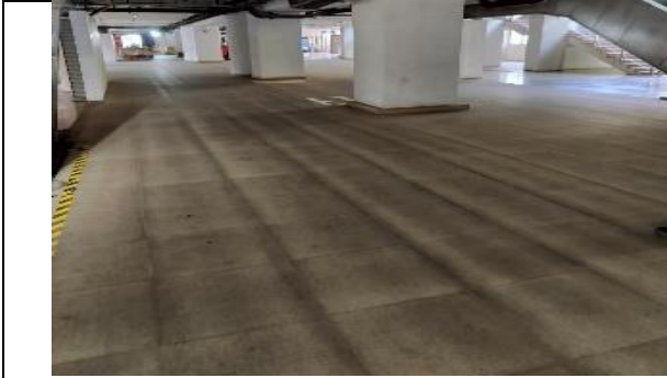
New Flooring provided to the Concourse Level after the CMRS Inspection
