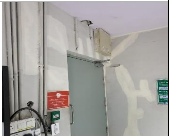
SCR room crack rectification work before CMRS inspection
